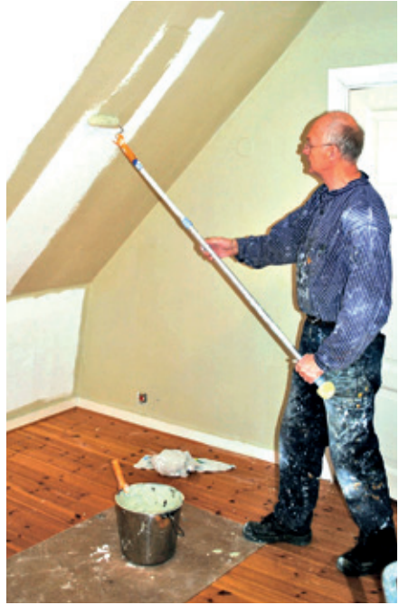
Painting papered walls with a roller.
