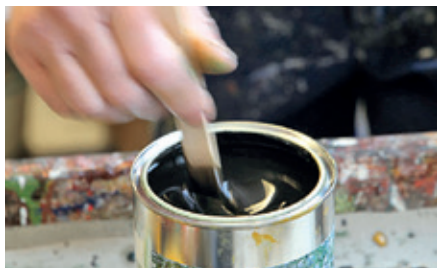
Stir the paint thoroughly before painting.
