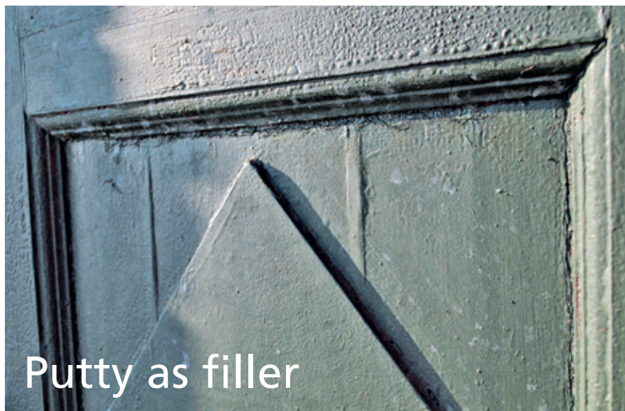
20 years after a simple "delay aging" measure with Linseed Putty in cracks and overpainting old, blistered linseed oil paint.
