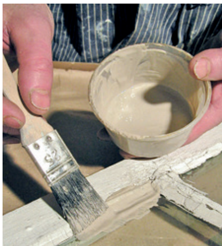
Thinned putty, a simple "delay aging" method.
